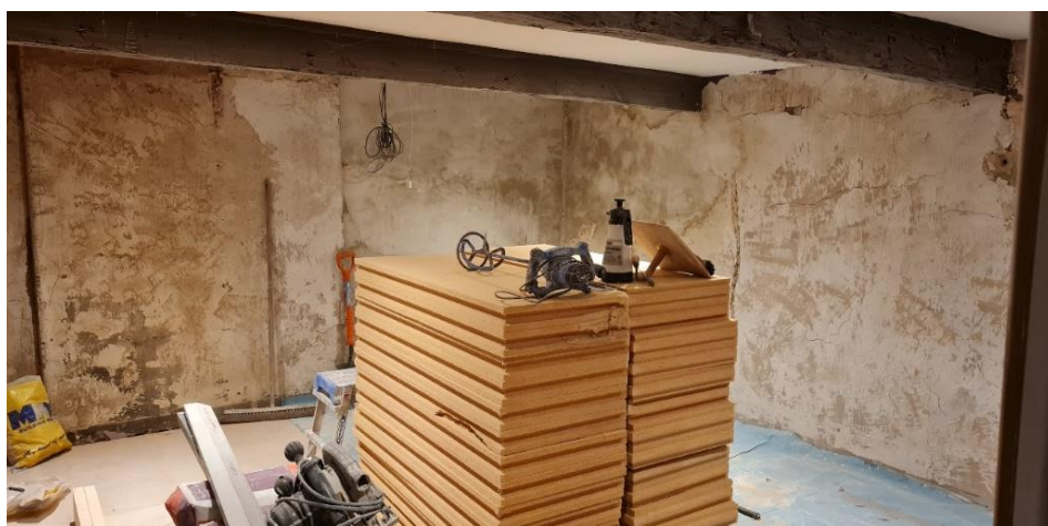
Bare walls before lining with special breathable insulation boards
